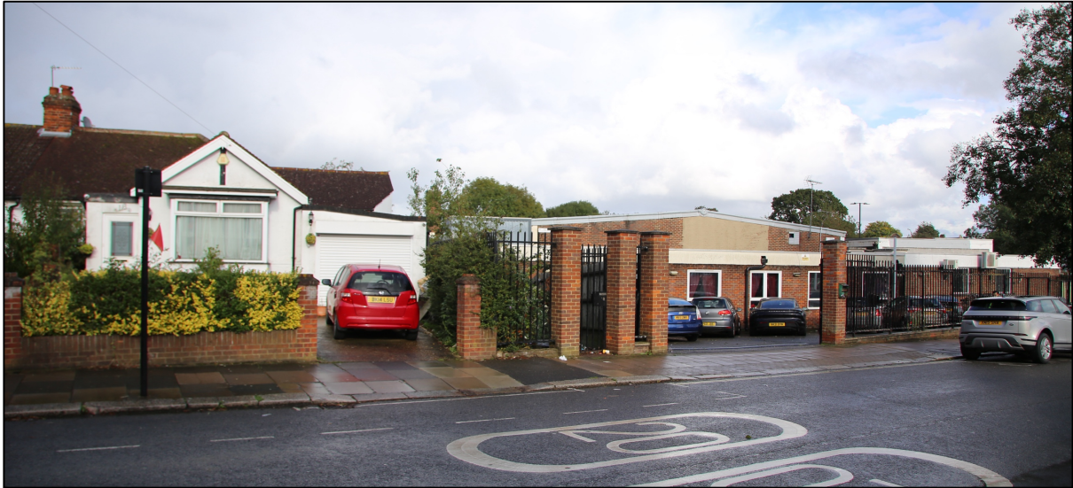
Existing view from Eastcote Lane
